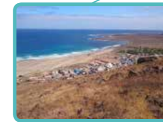
Cape Verde Municipal Water Supply
