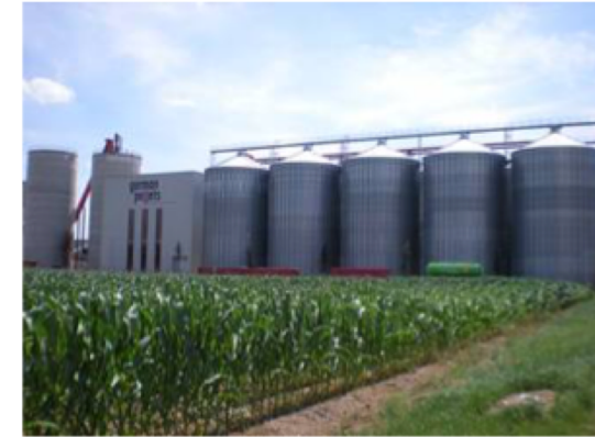
Pellet Storage Silos
