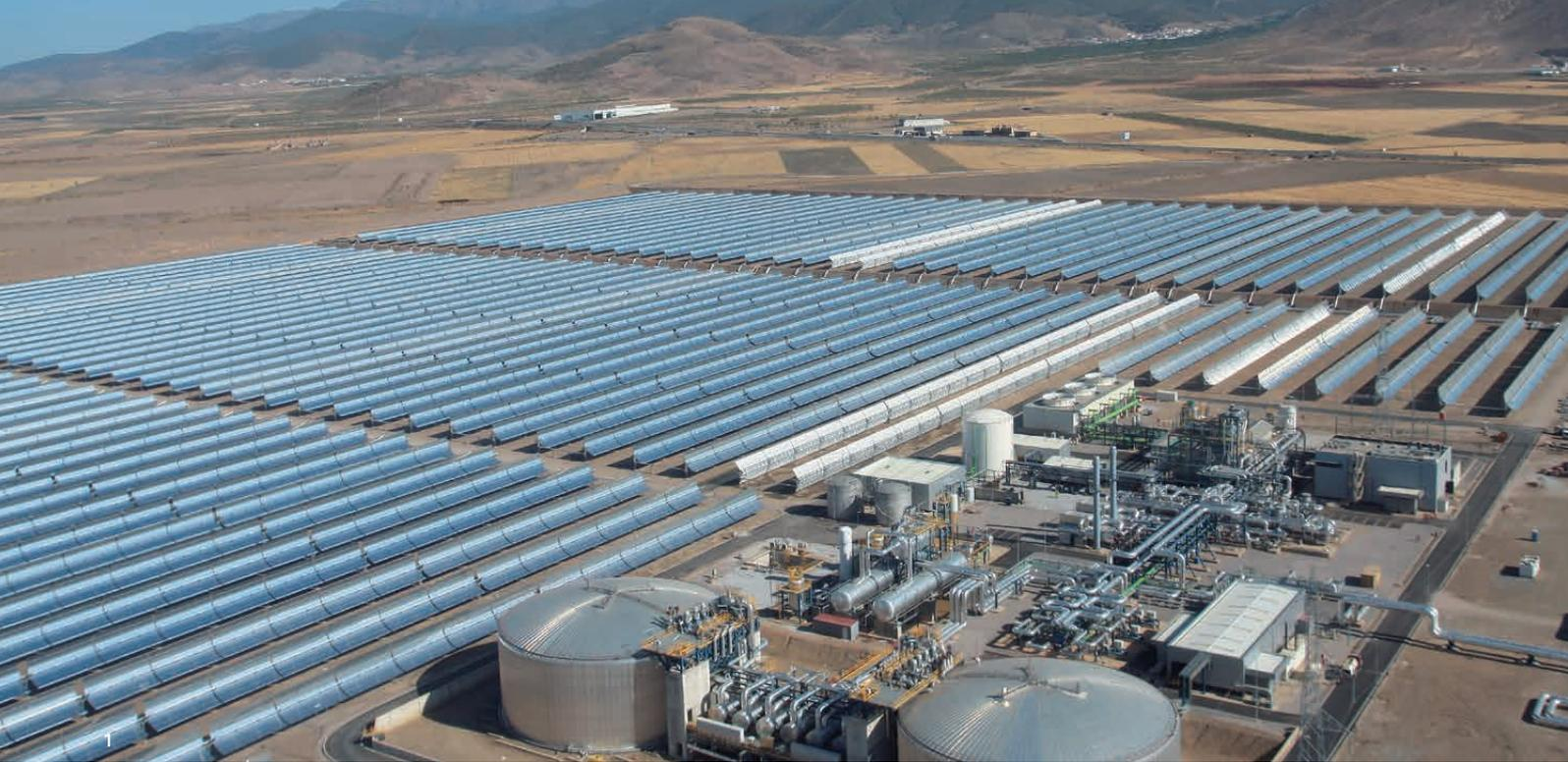
**Storage** In this context, solar thermal power plants represent an important option: in contrast to technologies like PV and Wind power, the thermal storage facilities of solar thermal power plants facilitate a demand-based supply of electricity comparable to that of fossil power plants, but based on the sun as a renewable fluctuating source of energy. Storage facilities are already capable of making electric power generation predictable and controllable (**Fig. 3**).
