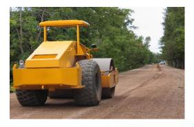
**4.** Compact and cap the road with topping materials, making sure to crown road for proper drainage.
