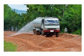
**2.** Add ECOROADS to the water truck and spray ECOROADS water solution onto the road base and windrow, as you would to bring soil to optimum moisture for compaction.
