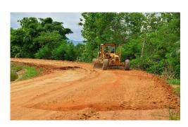
**1.** Grade the road according to the road design specifications desired, placing graded material to the side in a windrow.
