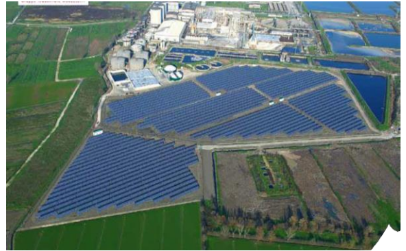
Location: Trecasali, Italy, 6MW Phono Solar
