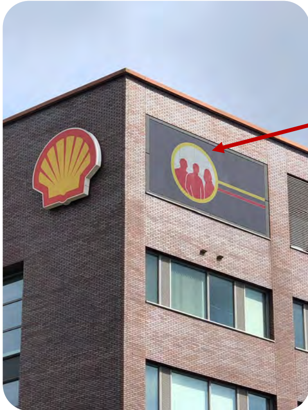
Shell design based on Star pattern Basic print coverage 30 % Energy yield 126 Wp/m 2
