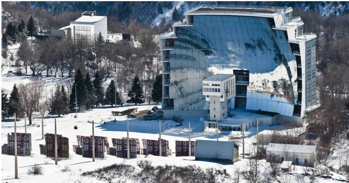
To replace the heat used by fossil fuels in industrial processes, researchers test solar thermal reactor designs at the PROMES testing lab at Odeillo in the French Pyrenees, capable of temperatures of up to 3,000°C IMAGE @ Sascha Burkhardt
