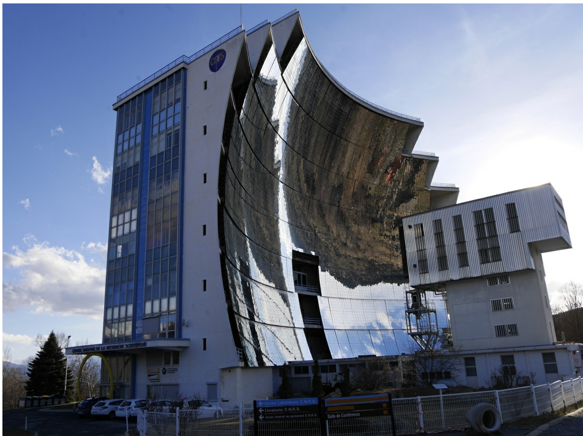
At the PROMES testing site in Odeillo, any temperature range can be tested. "For example, we were able to test our system here at lab bench scale and now we can test it at pilot scale in the same facility," Flamant explained. "PROMES is adaptable to a large range of solar flux, we can obtain a temperature higher than 3,000°C. IMAGE@PROMES
