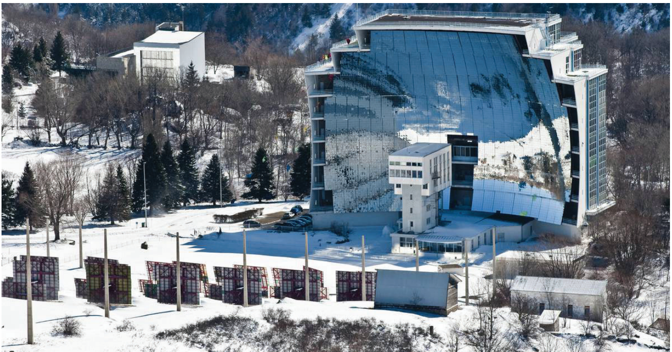
CNRS-PROMES solar furnace
