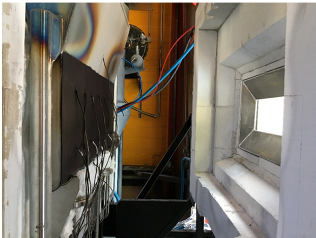
Fig. 6. View of the reactor (left) inside the cavity with the welded thermocouple on the front wall. Right side is the water-cooled aperture and the inner insulation.
