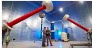
Low, Medium and High Voltage Electrical Equipment Assessment
