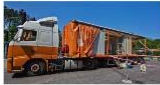
On-Site Commissioning, Diagnosis and Maintenance Tests of Electrical Equipment
