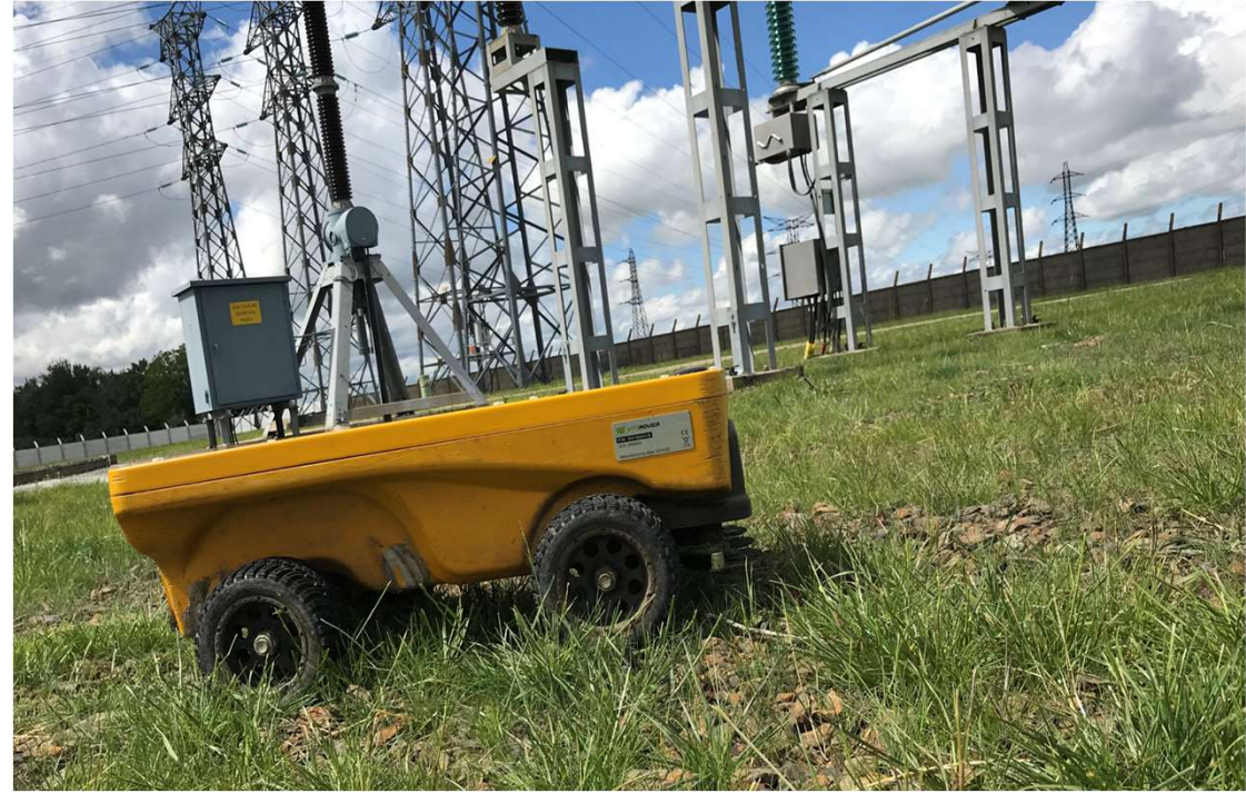
HIGHT VOLTAGE TRANSFORMERS
